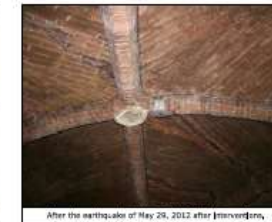
After the earthquake of May 29, 2012 after Interventions
